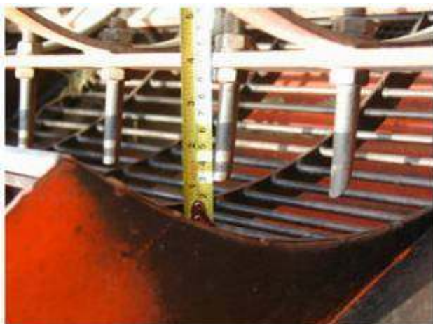
Figure 19: Checking the concave clearance
