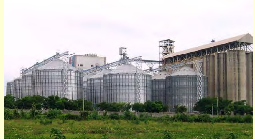
Concrete and steel silos
