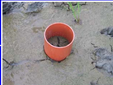
Appearance of installed PW tube
